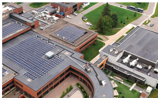
▲ Large-scale electric heat pump and thermal storage facility at Confederation College—the first of its kind in Northwestern Ontario.
